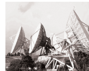
通信设备 Communication Equipment
